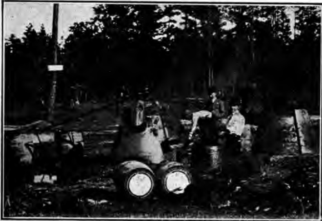
Fig. 14. Distilling Stumps in Place
